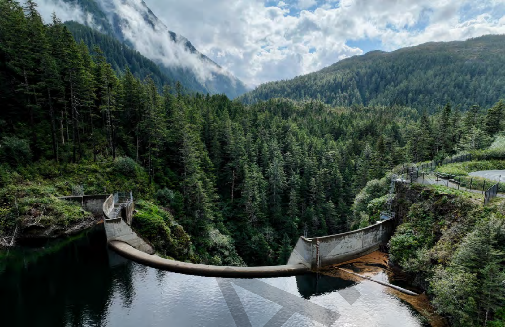
The backside of the Blue Lake dam
