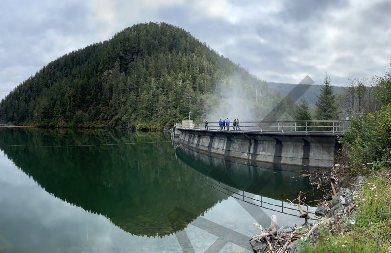
The backside of the Green Lake dam
