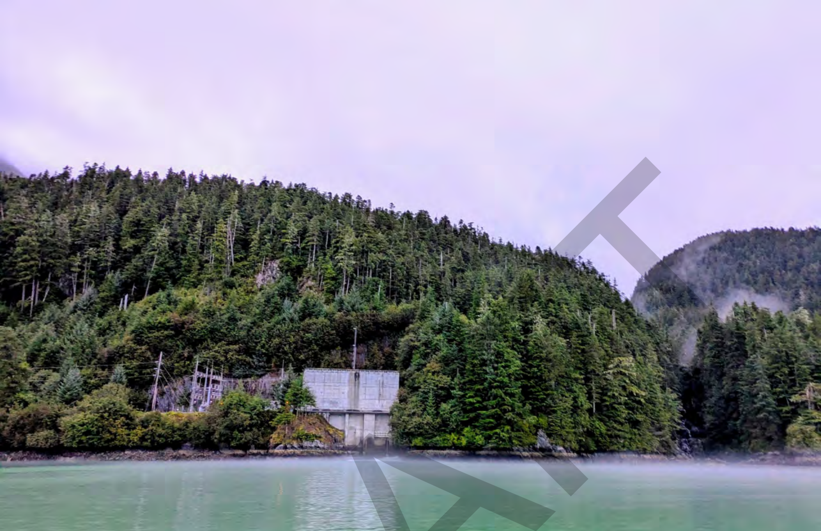
The Green Lake powerhouse on Silver Bay
