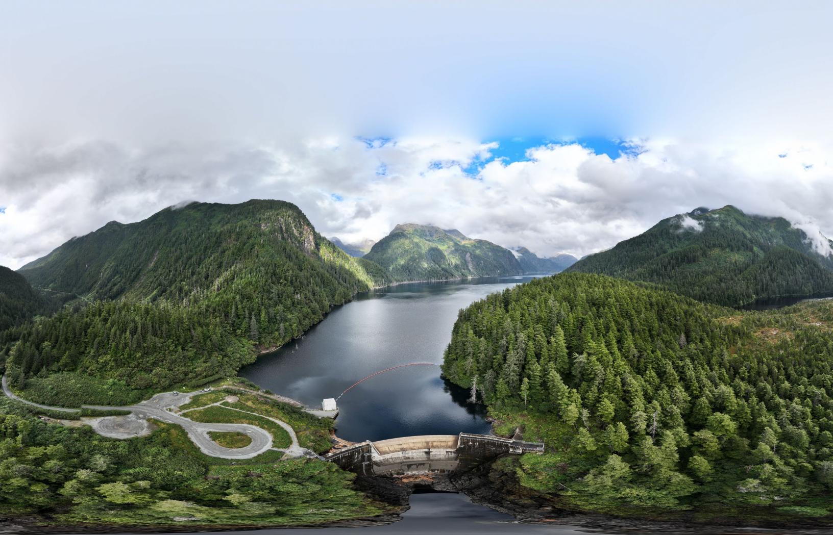
Panorama of the Blue Lake Hydroelectric Project
