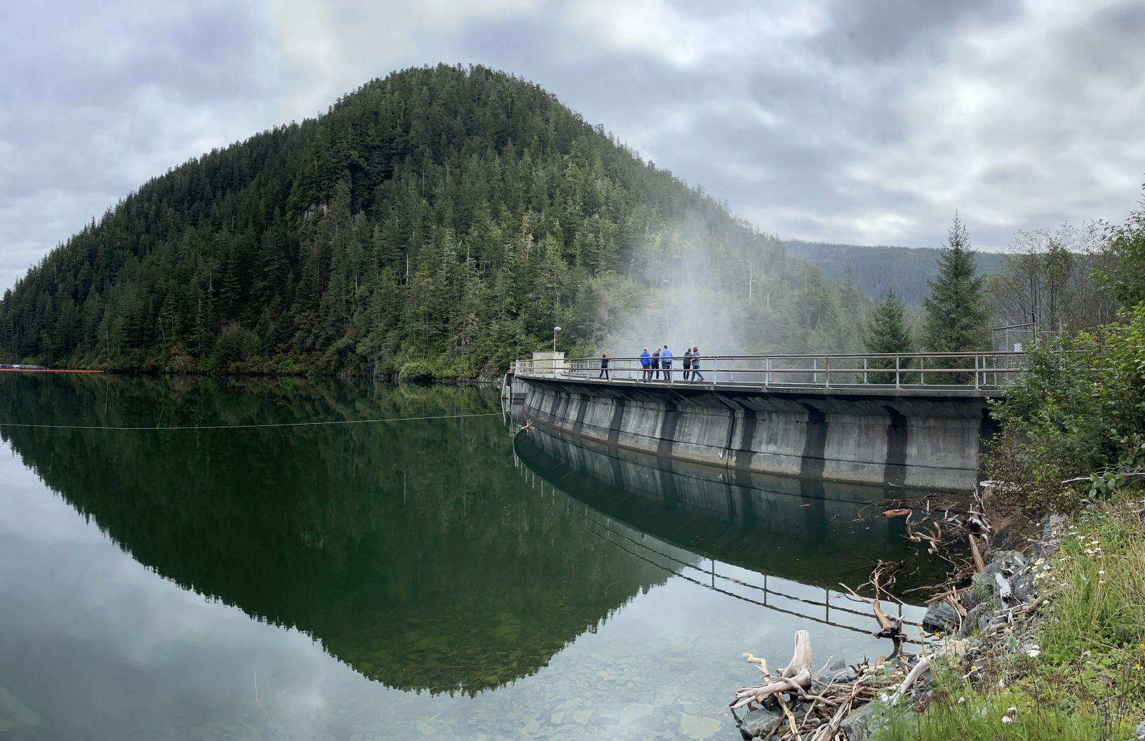
The backside of the Green Lake dam
