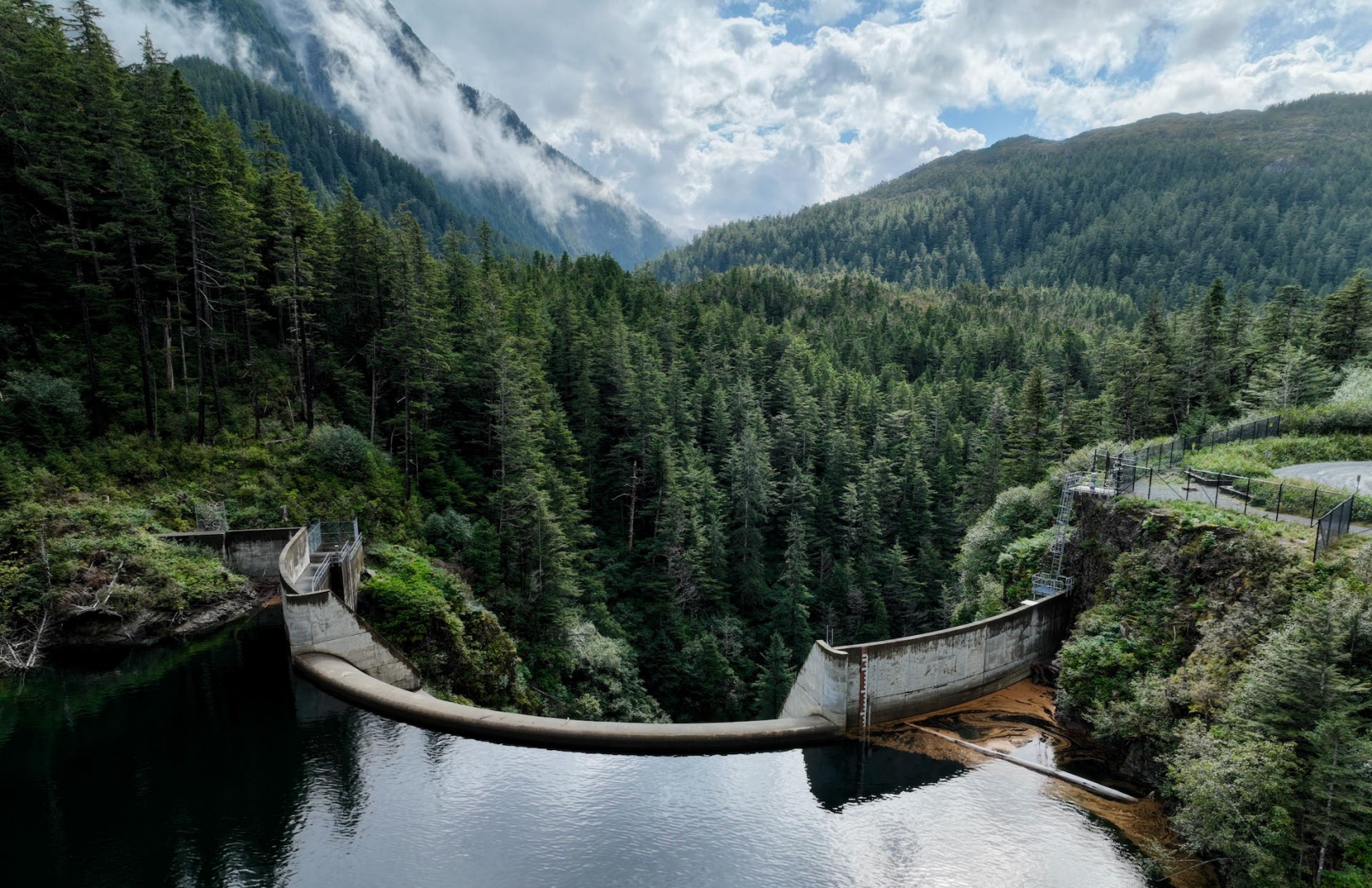
The backside of the Blue Lake dam
