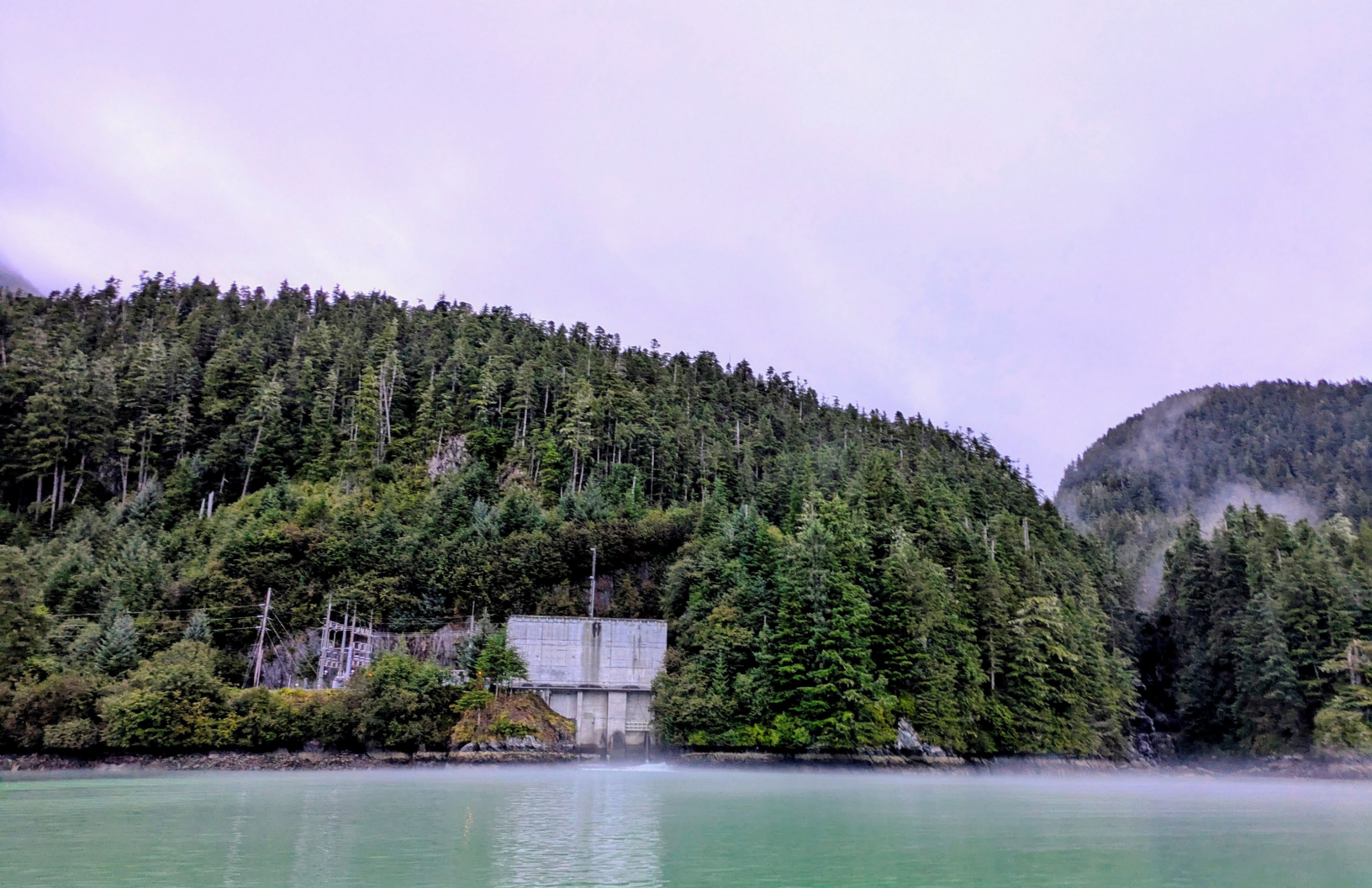
The Green Lake powerhouse on Silver Bay
