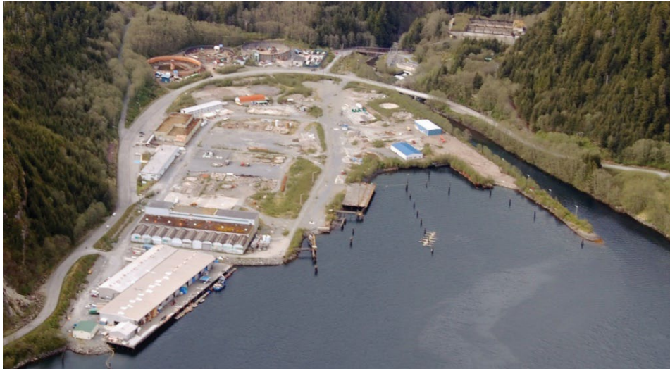
Figure 21. Gary Paxton Industrial Park Site in Early Development Stage
